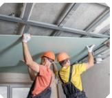
**Preassemble fixtures** or whatever you are fitting before installing them to minimize time spent working overhead.
